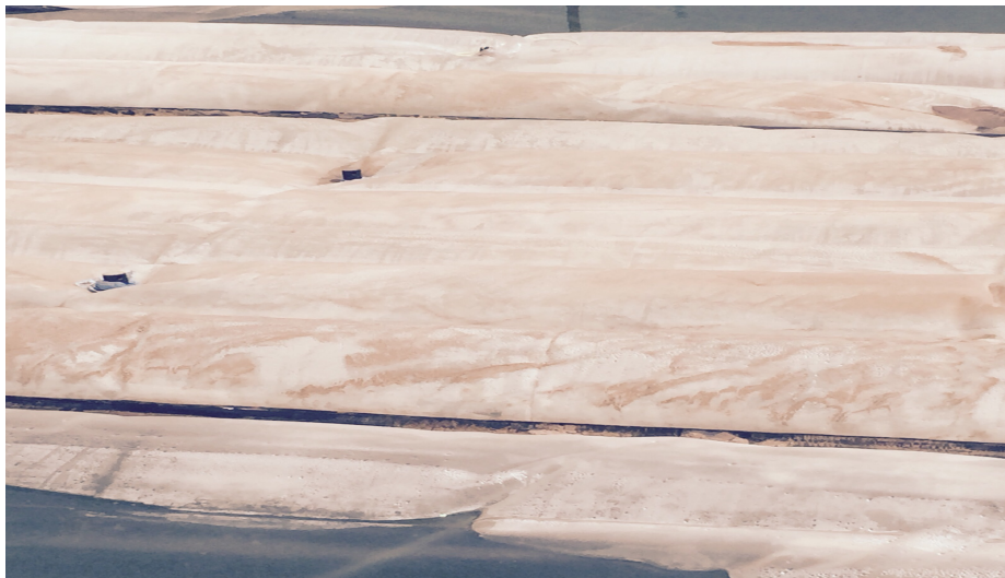
Figure 04.14 - Deterioration of the solar pond cover after a few weeks.
