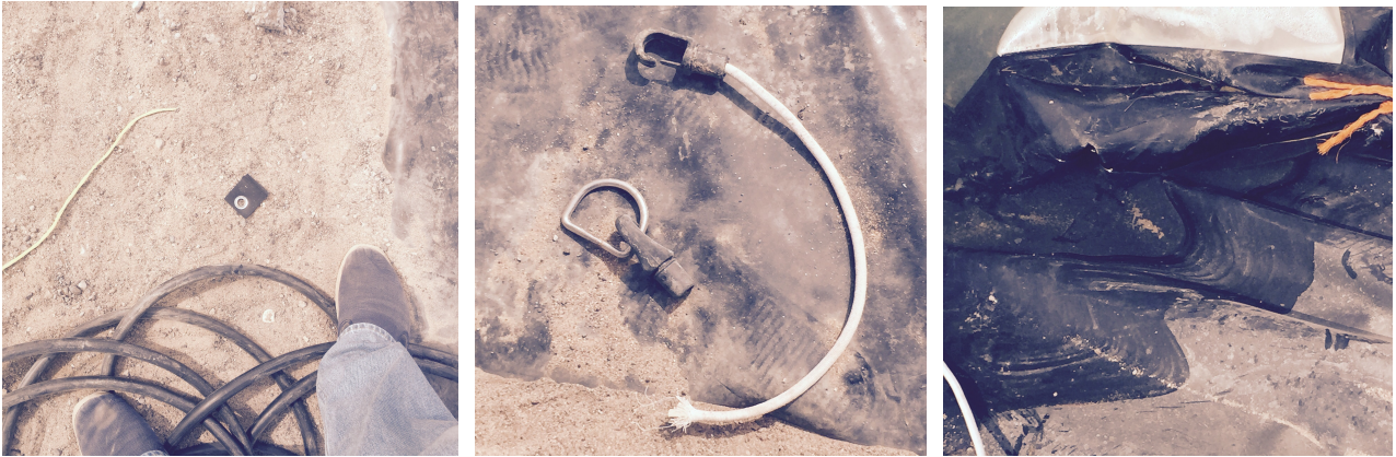
Figure 04.12 - Broken fixing parts during installation process.
