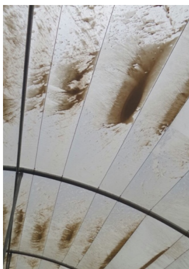
Figure 05.78 - Gypsum protective layer over the sheets of the greenhouse - Stage II/Part II.
