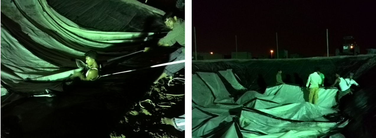
Figure 04.10 - SP installation over-night to avoid heat and hot surfaces.
