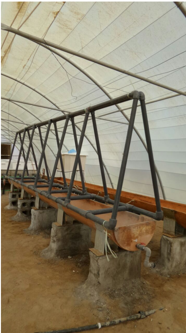
Figure 05.75: Frame structure of Prototype A (tent inside the greenhouse).
