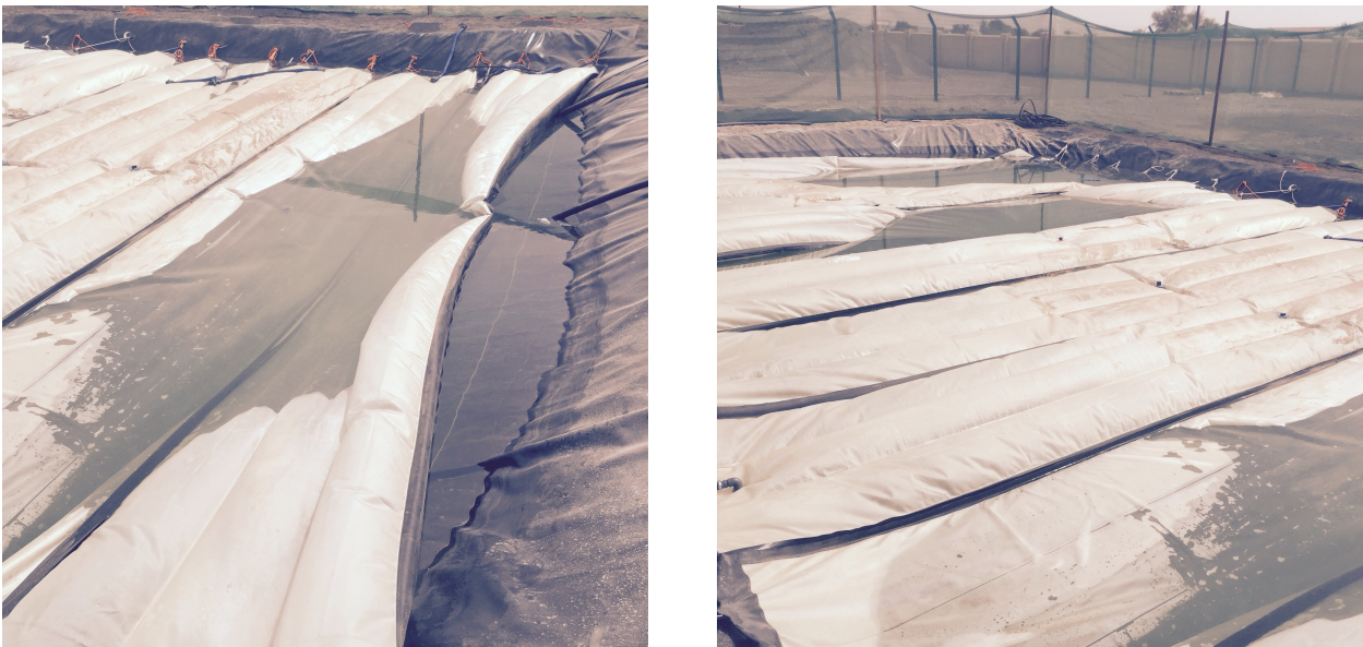
Figure 04.13 - Installation of the upper cover.
